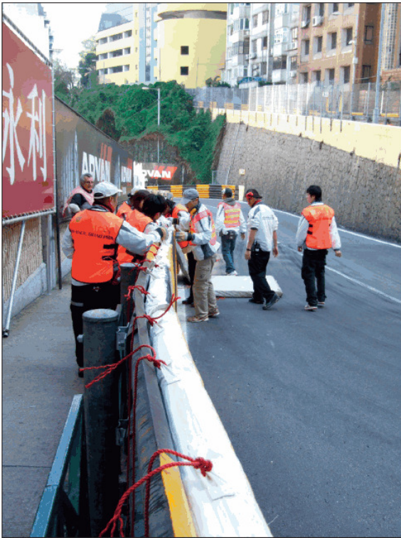
(Above) Workers tied rudimentary foam pads onto steel barriers before each on-course session for motorcycle racers. (Below, Right) Spectators pack a covered grandstand to watch multiple races at the Macau Grand Prix.
